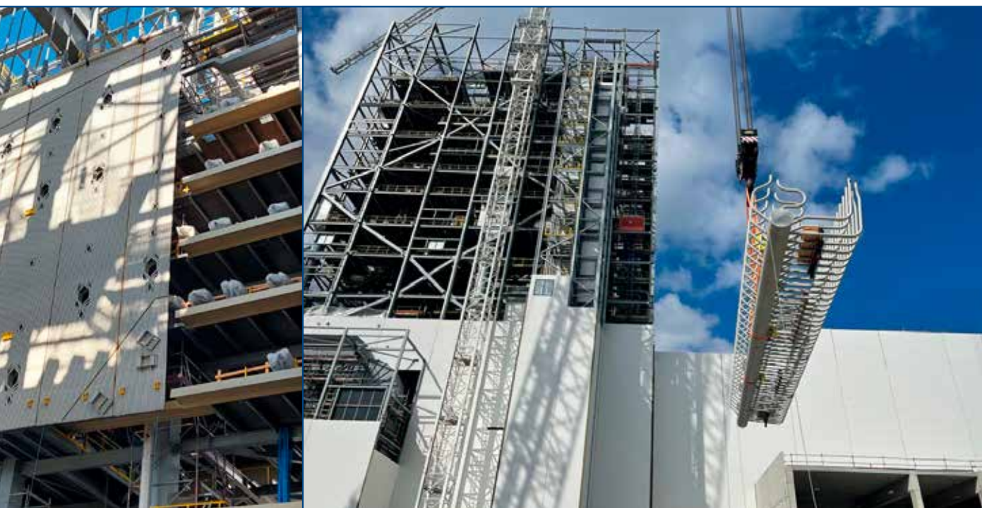
Kemi. Mechanical installation of an 8000 tds/d recovery boiler within the construction of a new bio-based paper mill. The complete plant of the new paper mill will produce approximately 1.5 million tons of softwood and hardwood pulp per year.
